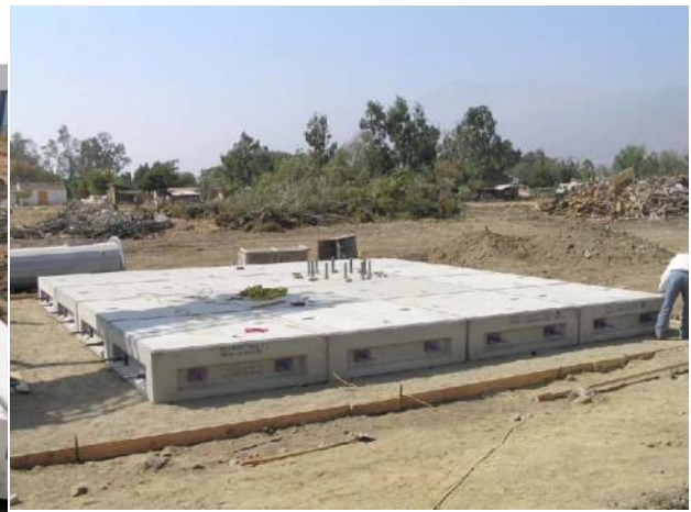
Figure 9: Precast slab foundation Source: Oldcastle precast, Inc.
