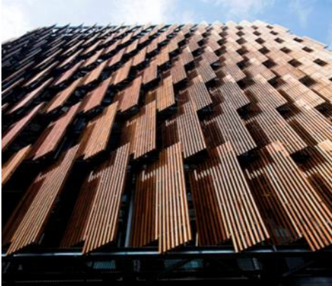
Figure 28: CH2 project, Melbourne, Australia : Recycled timber for façade screens of 10 storey high rise building, Source: www.nullabortimber.au
