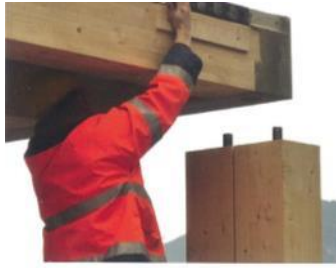
Figure 49: Assembly of ceiling element
