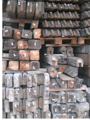
Figure 22: Storage of single elements and components of dismantled peat barn.
