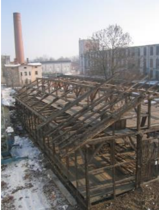
Figure 21: Existing peat barn in Kolbermoor, Germany, during dismantling phase.
