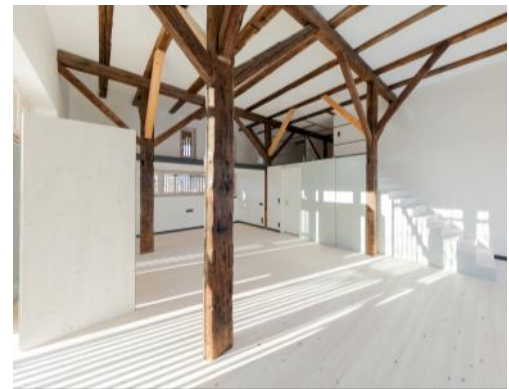
Figure 27: Finalised flat at ground floor level with historic structural system and modern elements for interior fit-out
