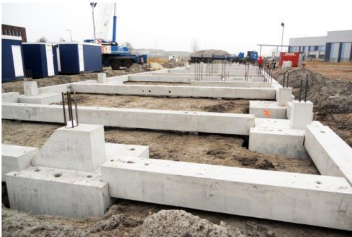
Figure 8: Vroom Precast strip foundation Source: Vroom Foundation Technology, NL
