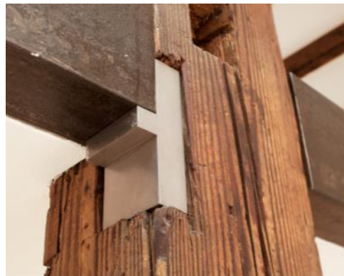
Figure 26: Historic beam with modern metal bearing for structural support of new crossbar
