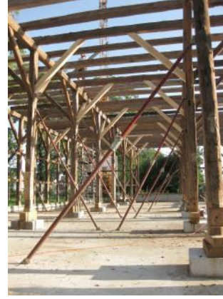
Figure 23: Reconstruction of support structure (columns and beams) on new foundations.
