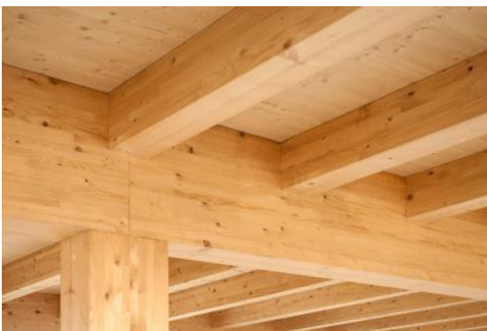
Figure 43: Solid timber beam from BSH
