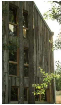
Figure 19: Reused timber for façade cladding, Source: www.nullabortimber.au
