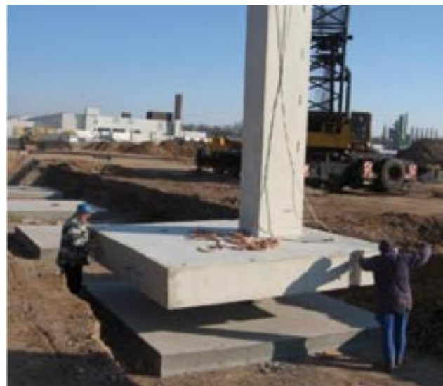
Figure 7: Column with cast-on foundation
