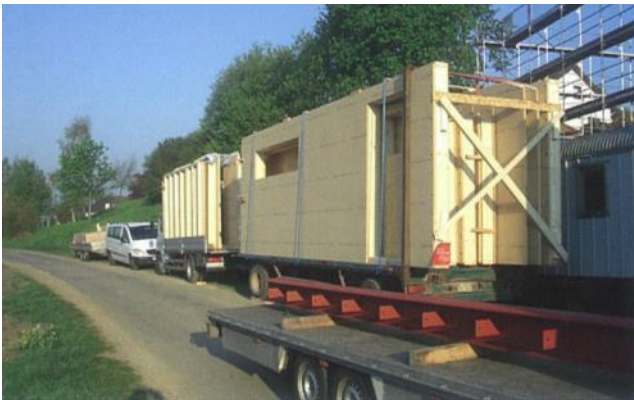
Figure 36: Transport of timber frame element, Source: Benedikt Wagner, Holzbau Schenk GmbH
