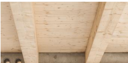
Figure 45: Solid timber ceiling from wood beams
