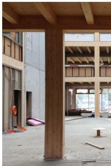
Figure 42: Solid timber column from BSH timber
