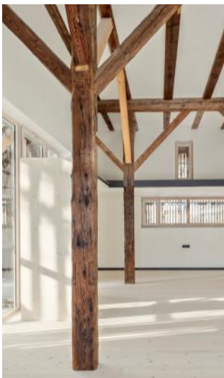
Figure 41: Solid timber column from one stem
