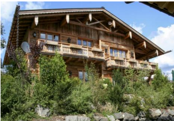
Figure 18: Reused timber from historic building for new construction of residential building, Source: www.Altholz.net
