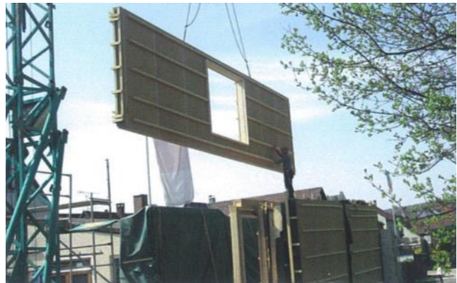
Figure 37: Assembly of timber frame element, Source: Frank Schäfer, 2-box Architekten
