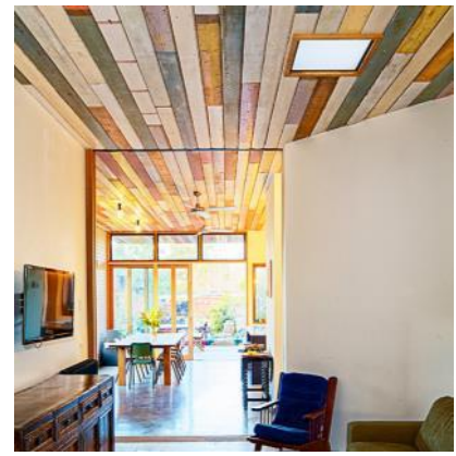
Figure 20: Reused timber as ceiling boards for a renovation project in Seddon, Australia, Source: www.sanctuarymagazine.org.au
