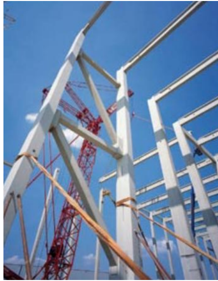
Figure 15: Bracing truss with precast concrete elements
