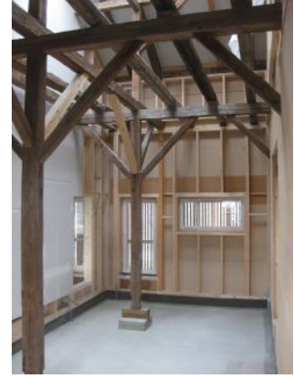
Figure 24: Historic support structure with internal partition walls from new materials.
