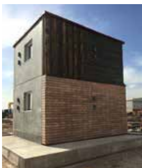
RE 4 BUILDING (SPAIN)
