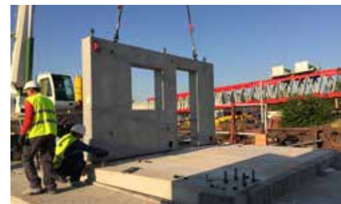
LOAD BEARING PREFABRICATED RE 4 PANEL WITH CDW
