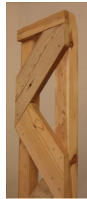
Figure 13. Framework studs, batters with different or same sizes, assembled eccentrically
