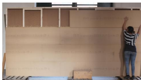
Figure 16. Application of wood fibre boards
