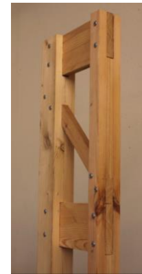
Figure 14. Framework stud, different sized batters, assembled centrally
