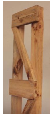
Figure 13. Framework studs, batters with different or same sizes, assembled eccentrically
