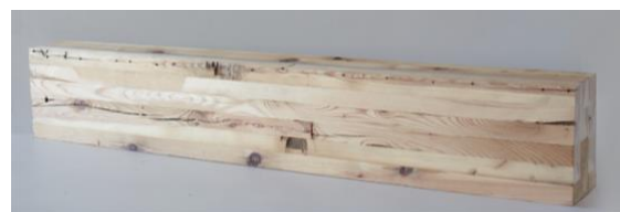
Figure 7. Glulam timber beam, with lamellas joined in vertical and horizontal direction
