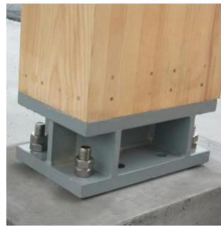
Figure 20. Bolted connection column - foundation
