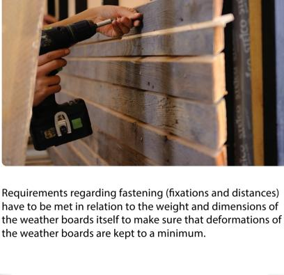
For the demonstration two different types of claddings are provided on the same façade element in order to test the weathering effect in relation to the orientation of the weatherboards.
