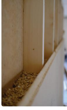
The hollow space in the manufactured panels was filled with a wood shaving insulation.
