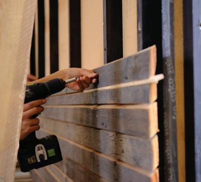
Requirements regarding fastening (fixations and distances) have to be met in relation to the weight and dimensions of the weather boards itself to make sure that deformations of the weather boards are kept to a minimum.
