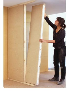
ZRS developed an innovative internal partition wall system which fosters the idea of prefabrication to enable easy installation and dismantling.
